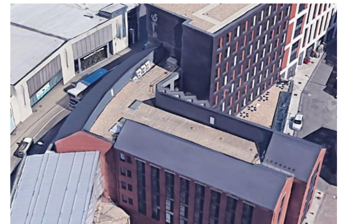
Image above: Good example of plant screening integrated into roof design
